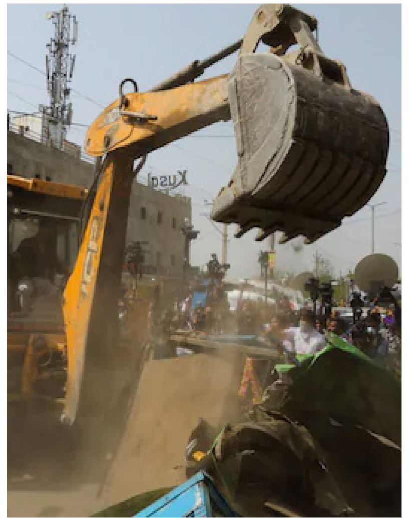
Demolition drive in Jahangirpuri
